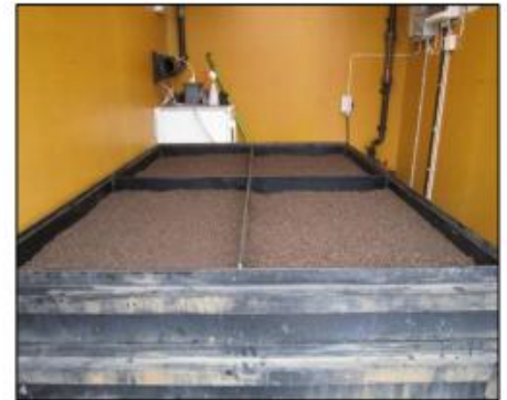
Aboveground Container-Housed Filter with Fresh Peat
