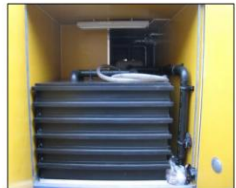
Aboveground Container-Housed Filter with Fresh Peat
